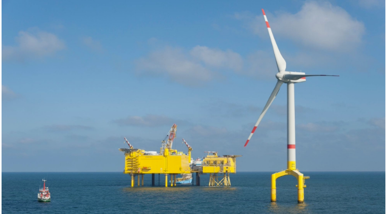
Image of BorWin Alpha and BorWin Beta Offshore Converter Station in the North Sea (TenneT 2024a, cited in NYSERDA 2025).
