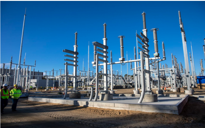
Onshore substation that receives power from Vineyard Wind 1 transmission cables ( Image: Robin Lubbock/WBUR, 2023 ).
