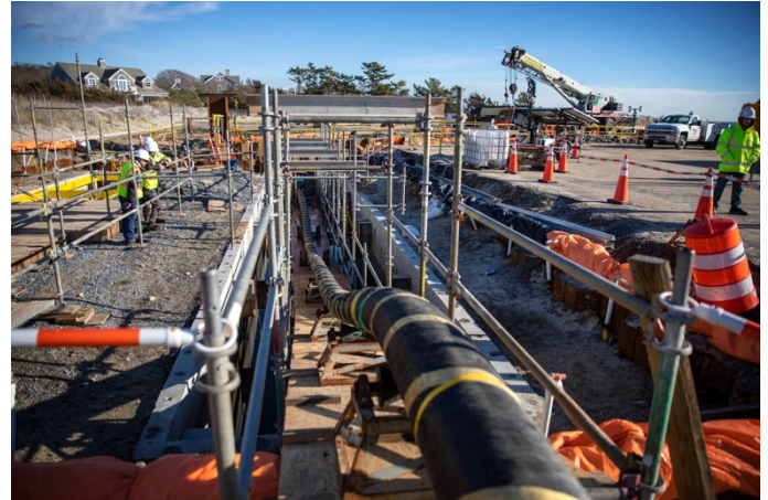
Offshore wind transmission cable from the Vineyard Wind 1 project in the transition joint bay ( Image: Robin Lubbock/WBUR, 2023 ).
